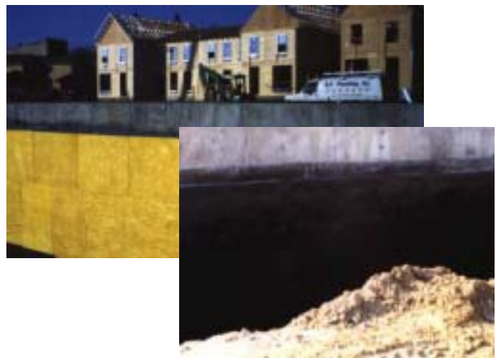
Typical spray application of System 17 PMA.
