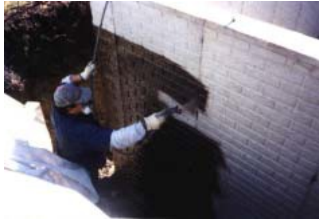
System 17 PMA forms a tough, durable finish which bridges shrinkage cracks.
